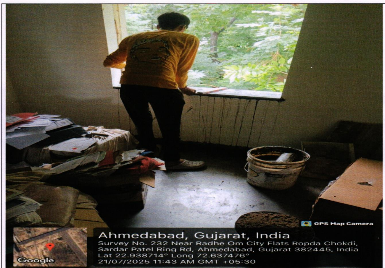
Civil work for window in progress
