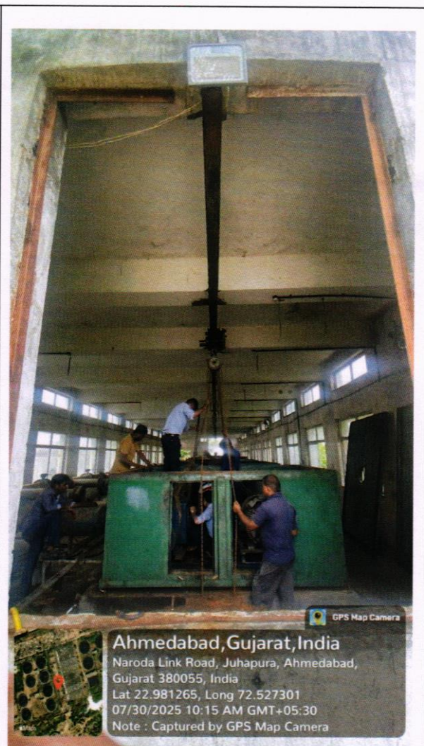
Repaired blower's installation work in progress at blower room
