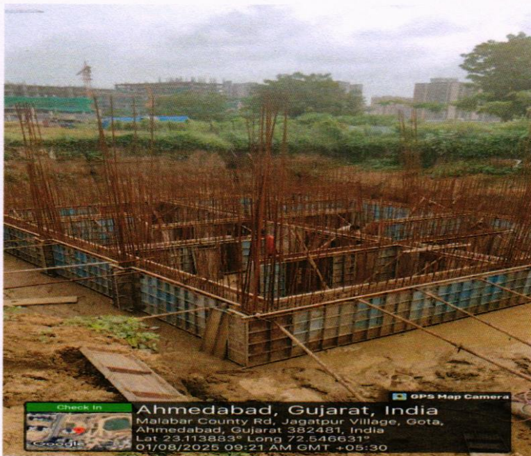
CCT 1 st Lift Shuttering
