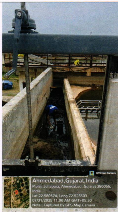
Bottom sludge cleaning work in progress at PTU for C-stream
