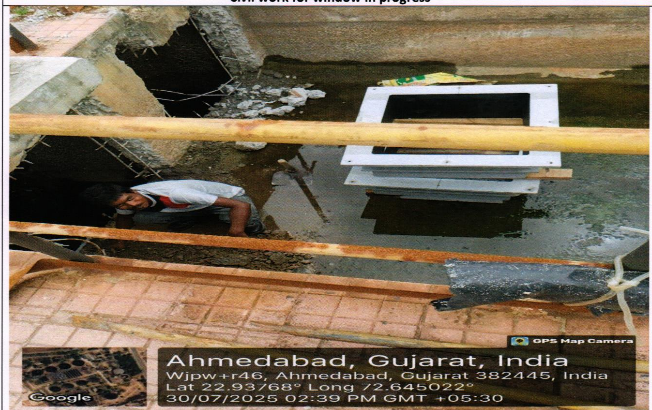
Gate installation in progress for stream-1
