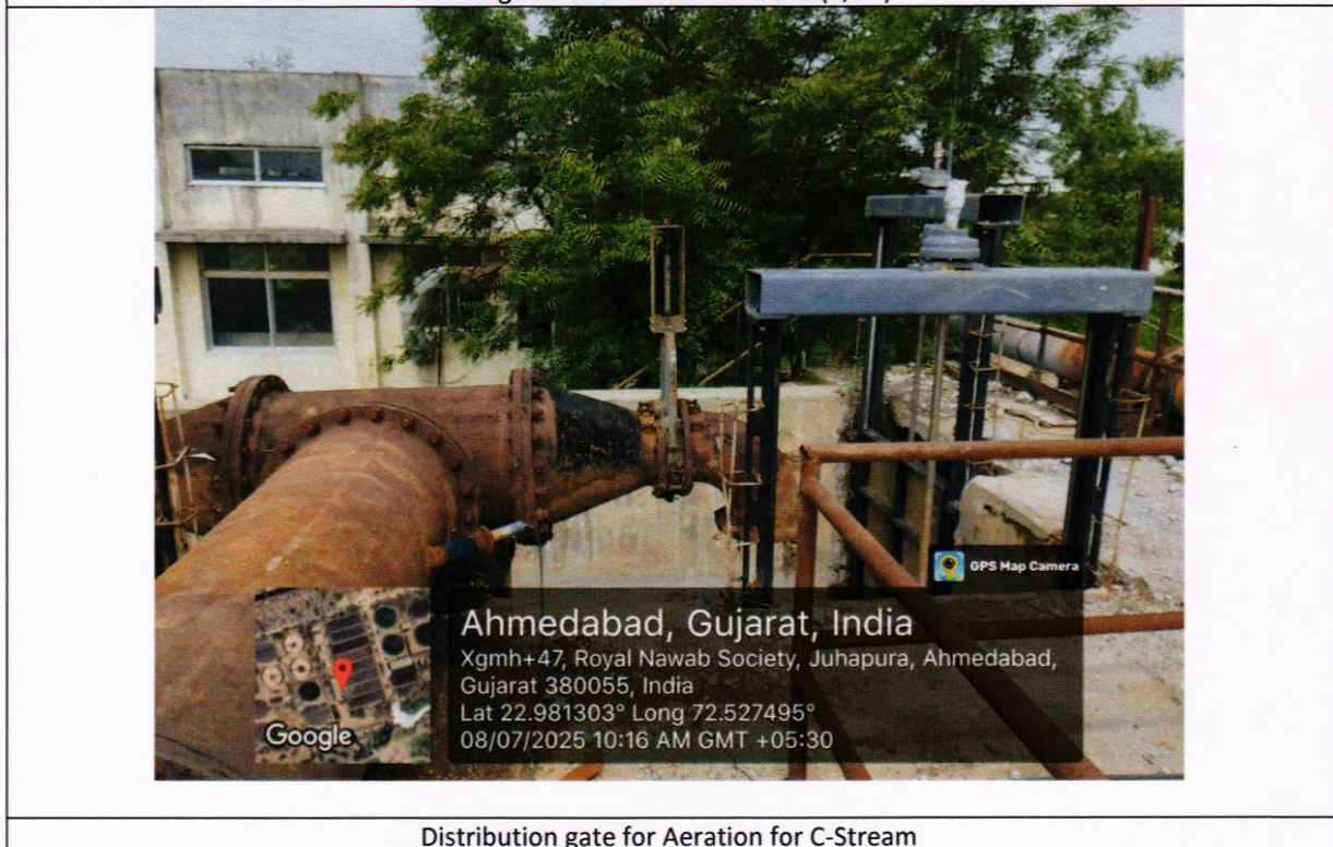
PTU gate installed for C- stream (7/10)
