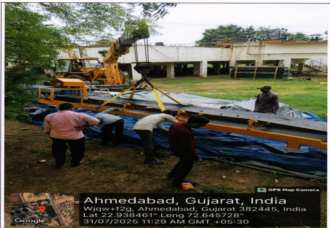
Belt conveyor Installation in progress
