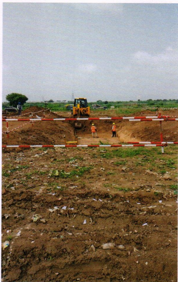
SBR EXCAVATION IN PROGRESS.
