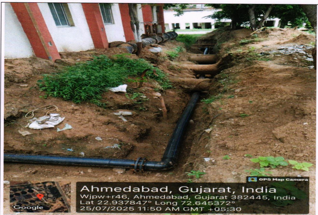
HDPE sludge line from thickner to thicken sludge pump house completed.
