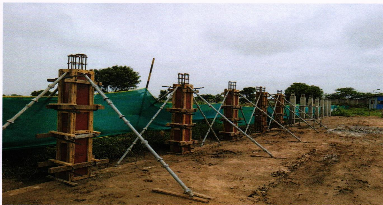
BOUDARY WALL CONSTRUCTION.
