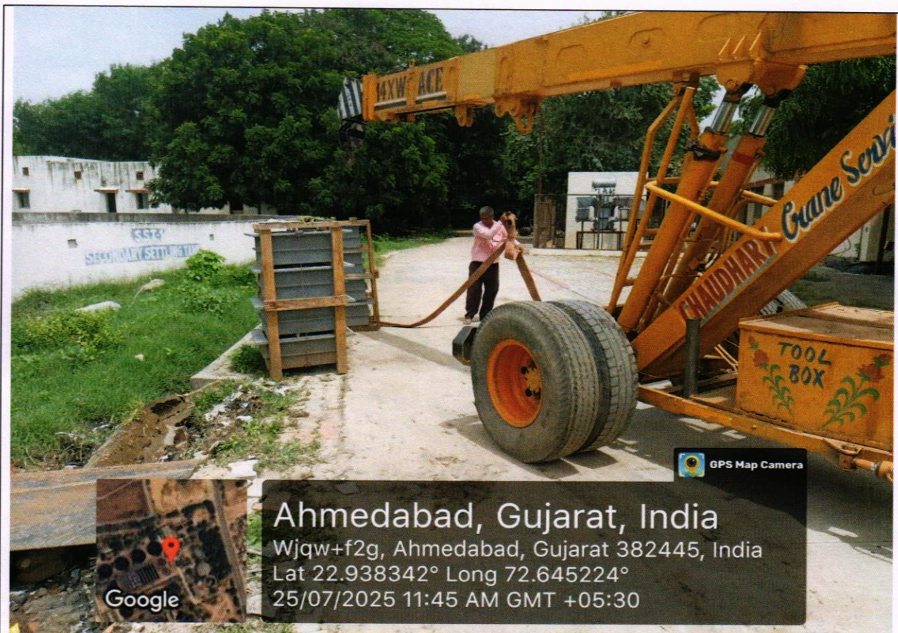
Gate installation in progress for stream-1
